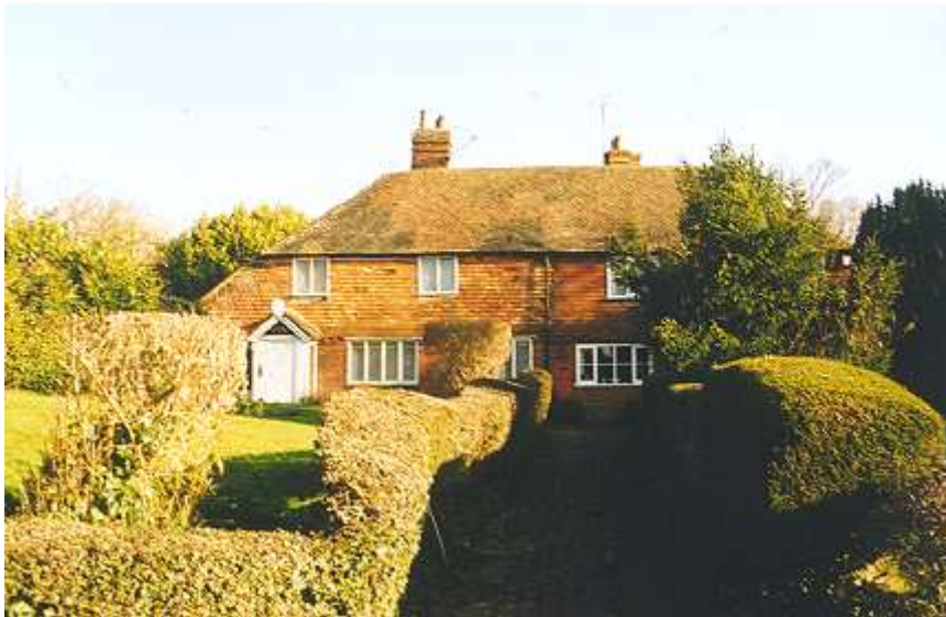
Figure 2 Post Office Cottage and the Old Post Office
