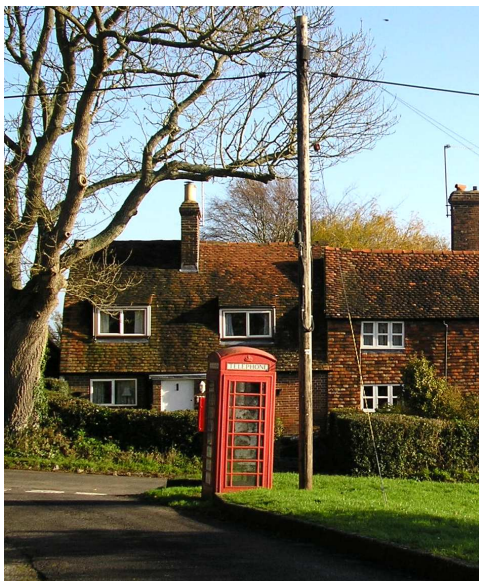
Figure 18 Prominent pole and overhead lines'
